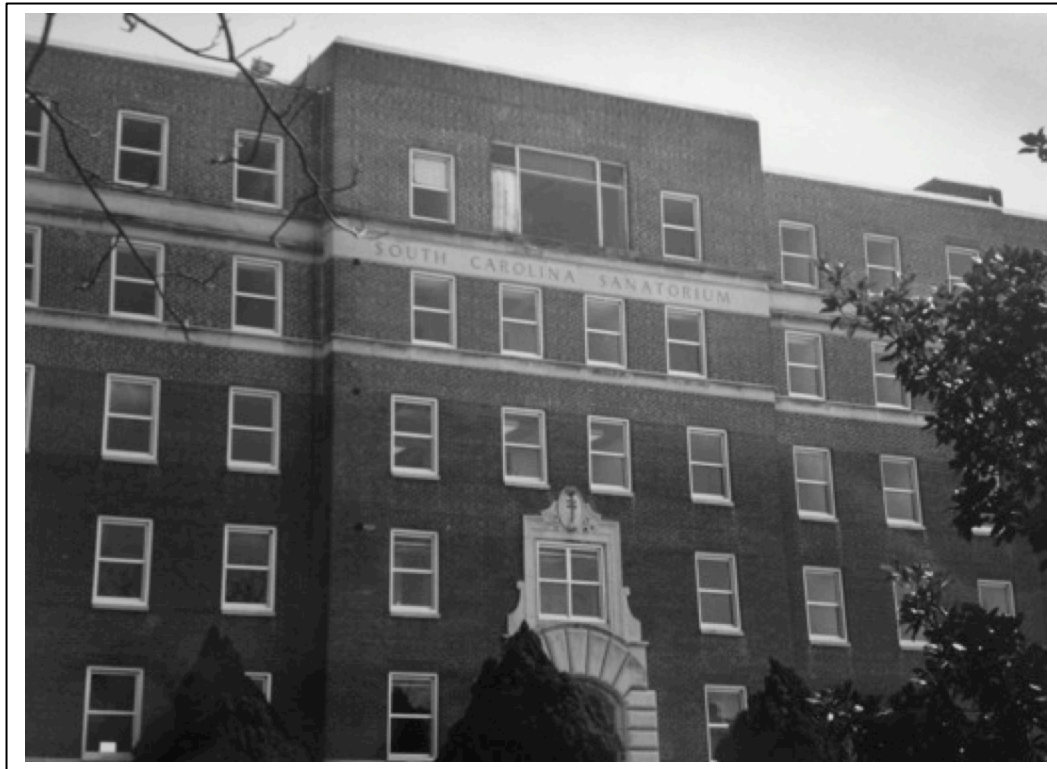
Figure 2.14 The PWA building was the first patient structure at the sanatorium built from brick. Fire hazard was a common concern of the administration, especially after a fire took place in a patient pavilion in 1932. Brick buildings were seen as improvements to the healthcare provided at the hospital. White patients were treated here after the completion of the PWA building, while black patients were segregated to the older, wooden structures on the property until the 1950s.
