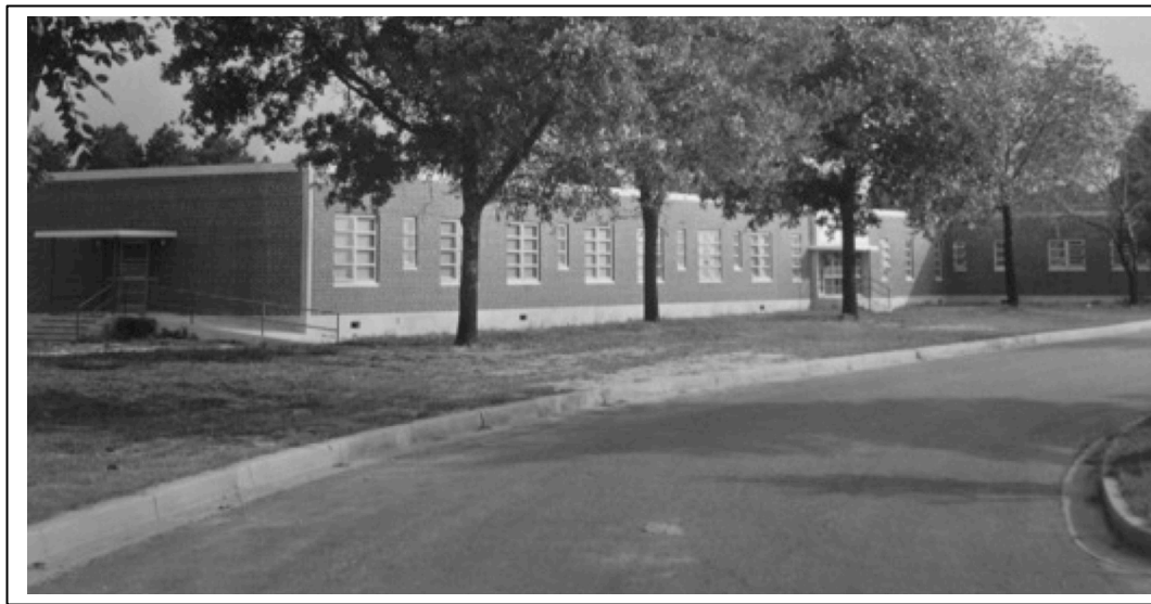
Figure 2.18 This low brick structure was built in 1954. The roof was reinforced to accommodate an additional floor if the sanatorium wanted to expand the facility. Unlike previous patient wards, this structure has no porches or sundecks. Antibiotics became widely used for tuberculosis treatment in the 1950s, reducing the medical need for these architectural elements.
