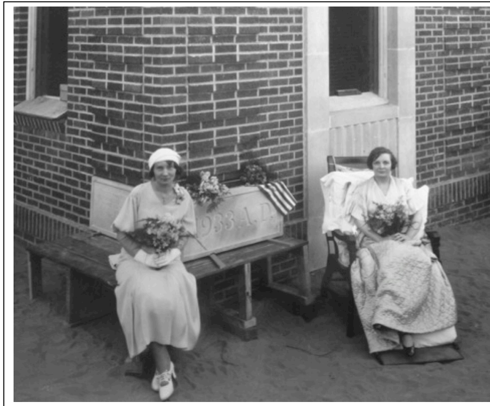
Figure 2.11 Patients contributed to the development of the sanatorium. Here, two women sit at the construction site of the Earnest Cooper Community Building in 1933. The pillows, blanket, and reclining chair, indicate the woman on the right is most likely a patient. Patients, and women in particular, played an essential role in funding and helping to design the Cooper Community Building.
