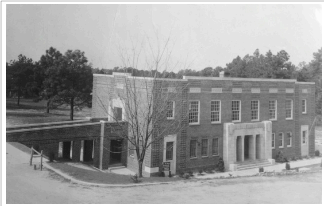
Figure 2.10 Note the ramp on the side of the Cooper Community Building. The ramp provided access to the second-story auditorium for patients too ill to use the interior stairs. Patients at the sanatorium conceived the idea for a community building and fundraised for ten years in order to make their vision a reality. Patients' needs, such as ramp access, are seen in the architectural design of the building.
